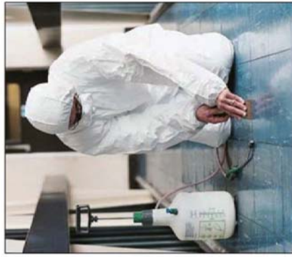
Spray water under the tiles to suppress dust as you lift them gently, avoiding breakage
